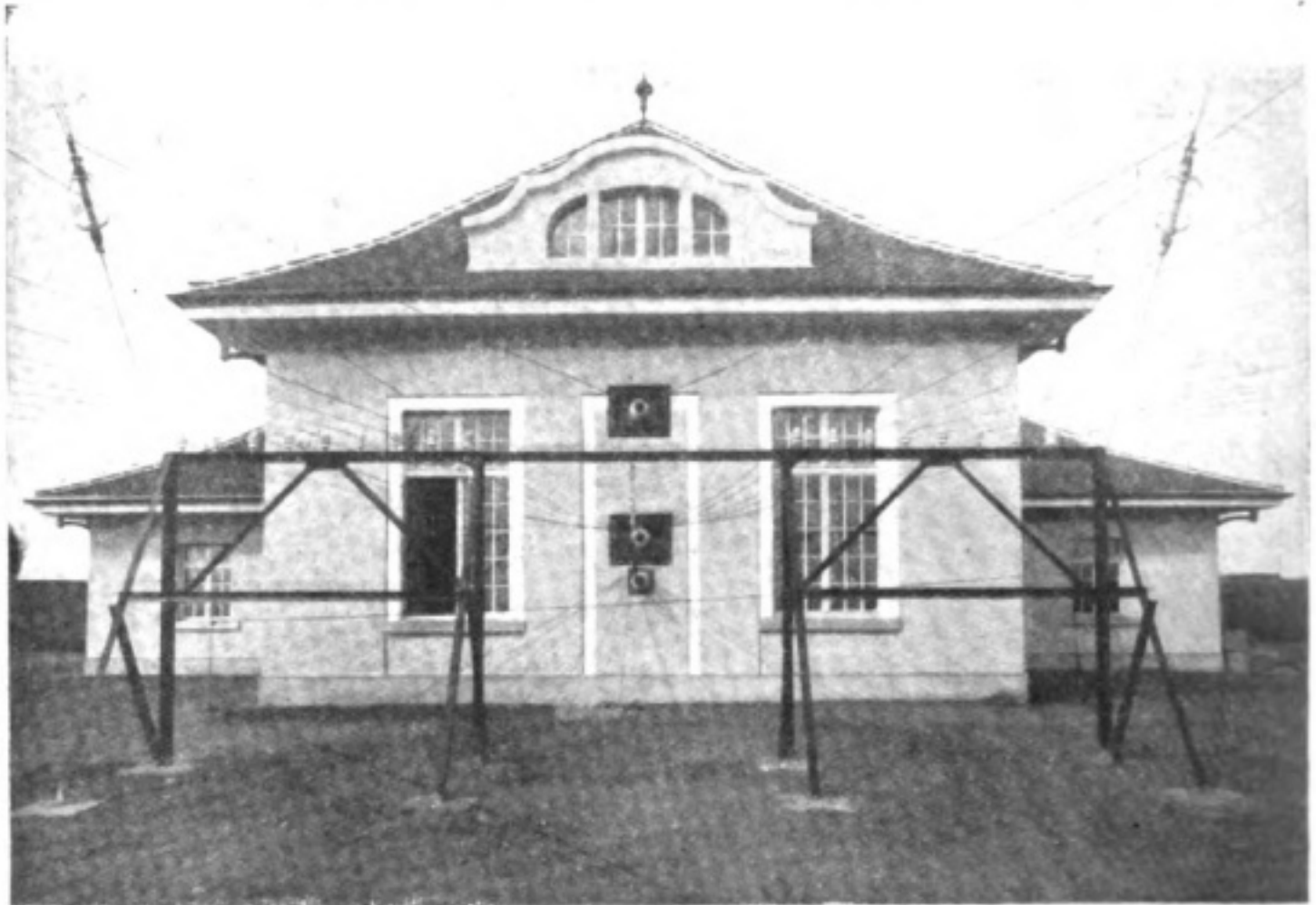
Berne Wireless Station. The "Leading-in" Insulators for Aerial and Earth Screen and Ordinary Ground Earth.
